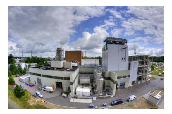
The bioliq plant at KIT: In a multi-stage process, high-quality synthetic fuels are produced from straw and other biogenous residues. Credit: KIT/Tom Zevaco
