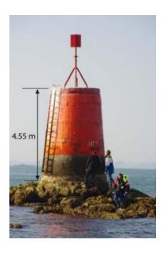
A lighthouse turret off the coast of Lorient in Brittany has been enhanced with technology developed at EPFL for bridges. This trial run will test the application of Ultra-High Performance Concrete (UHPC).
