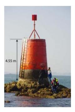
A lighthouse turret off the coast of Lorient in Brittany has been enhanced with technology developed at EPFL for bridges. This trial run will test the application of Ultra-High Performance Concrete (UHPC).
