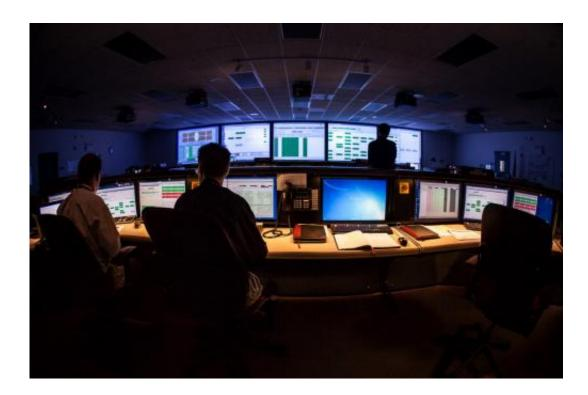
All NIF experiments are controlled and orchestrated by the integrated computer control system in the facility's control room. It consists of 300 front-end processors attached to about 60,000 control points, including mirrors, lenses, motors, sensors, cameras, amplifiers, capacitors and diagnostic instruments.
