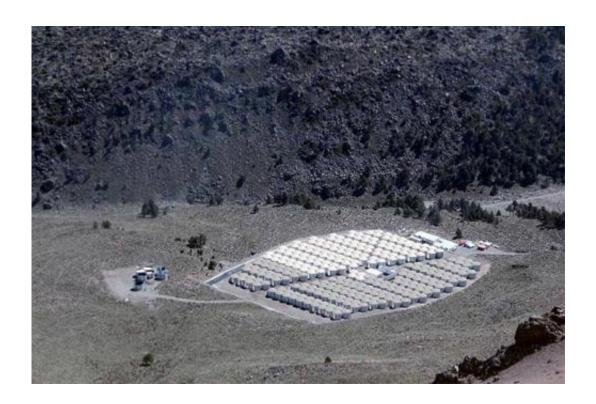
The HAWC Observatory taken in August 2013 from the summit of Sierra Negra. The image has been digitally altered to show HAWC as it will appear when construction is complete in 2014. The 111 Cherenkov detectors currently installed (100 Cherenkov detectors in operation) are colored white and located in the upper right quadrant of the array.
