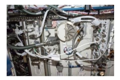
Amine Swingbed payload is shown during installation into EXPRESS Rack 8 during Expedition 35. EXPRESS is short for Expedite the Processing of Experiments to Space Station. Credit: NASA
