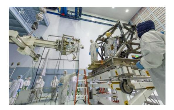
MIRI, the mid-infrared camera and spectrograph (left), was installed in the science payload module of the James Webb Space Telescope (right) on 29 April 2013 at the NASA Goddard Space Flight Center. Credit: NASA/C. Gunn
