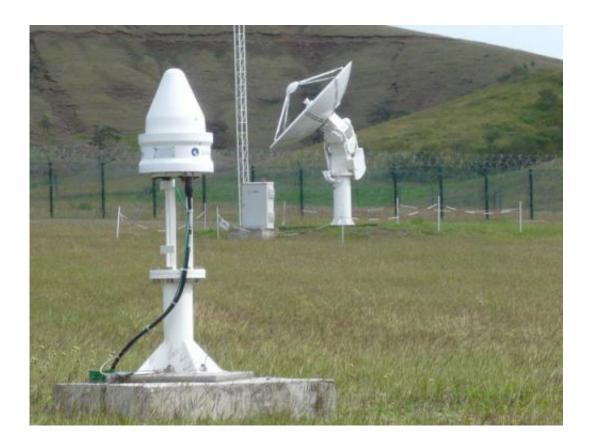
The Galileo ground station near New Caledonia capital Nouméa incorporates a Galileo Sensor Station (foreground) that monitors the quality of navigation signals and an Uplink Station (background) to relay navigation corrections to the satellites for rebroadcast to users. An antenna 13 m in diameter for controlling the satellites has also been built, ready to come online later this year. Credit: ESA-Fermin Alvarez Lopez
