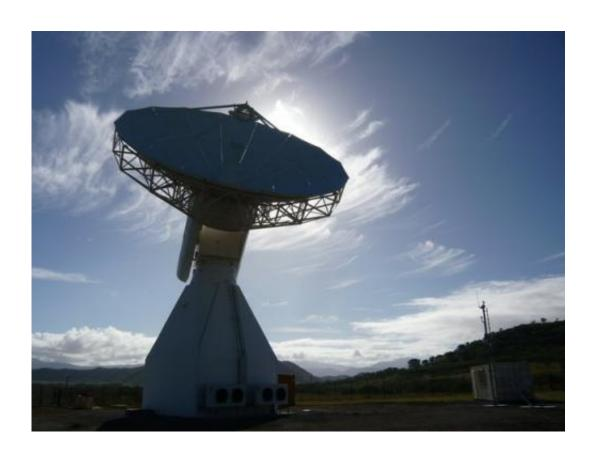
A 'telemetry, tracking and command' antenna, 13 m in diameter, for controlling Galileo satellites at the Galileo ground station near Nouméa, New Caledonia. The antenna is due to begin operations later in 2013. Part of a growing worldwide network, the ground station incorporates a Galileo Sensor Station that monitors the quality of navigation signals and an Uplink Station to relay navigation corrections to the satellites for rebroadcast to users. Credit: ESA - Fermin Alvarez Lopez
