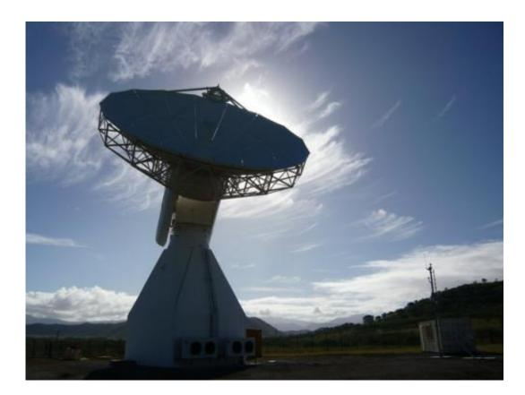
A 'telemetry, tracking and command' antenna, 13 m in diameter, for controlling Galileo satellites at the Galileo ground station near Nouméa, New Caledonia. The antenna is due to begin operations later in 2013. Part of a growing worldwide network, the ground station incorporates a Galileo Sensor Station that monitors the quality of navigation signals and an Uplink Station to relay navigation corrections to the satellites for rebroadcast to users. Credit: ESA -Fermin Alvarez Lopez
