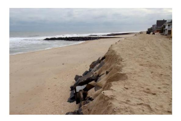
A forgotten, 1,260-meter seawall buried beneath the beach helped Bay Head weather Sandy's record storm surges and large waves over multiple high tides, according to a team of engineers and geoscientists led by Jennifer L. Irish, an authority on storm surge, tsunami inundation, and erosion at Virginia Tech. Credit: Jennifer Irish/Virginia Tech
