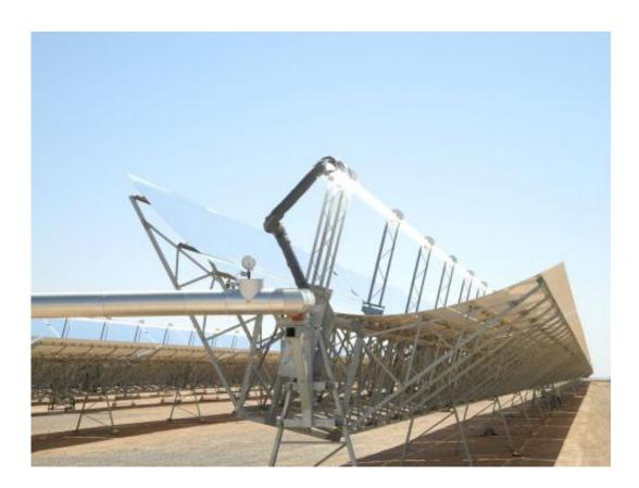
Concentrated solar power systems use mirrors or lenses to concentrate a large area of sunlight, or solar thermal energy, onto a small area. Credit: Dii / UNEP
