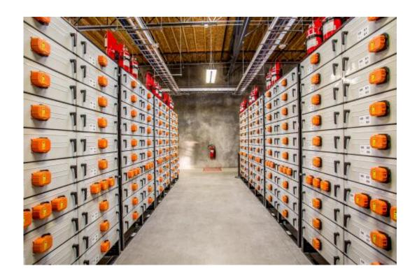
Rows of battery racks at Portland General Electric's Salem Smart Power Center in Salem, Ore. PGE is a participant in the Battelle-led Pacific Northwest Smart Grid Demonstration Project, which will use the center's 5-megawatt energy storage system to test several smart grid technologies and approaches. Credit: Portland General Electric
