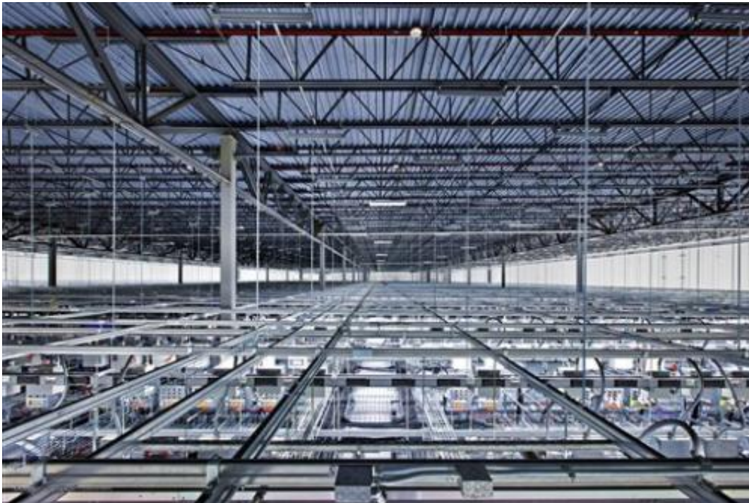
This undated photo made available by Google shows the view from the floor in Council Bluffs, Iowa. Huge steel beams both support the structure and help distribute power. (AP Photo/Google, Connie Zhou)
