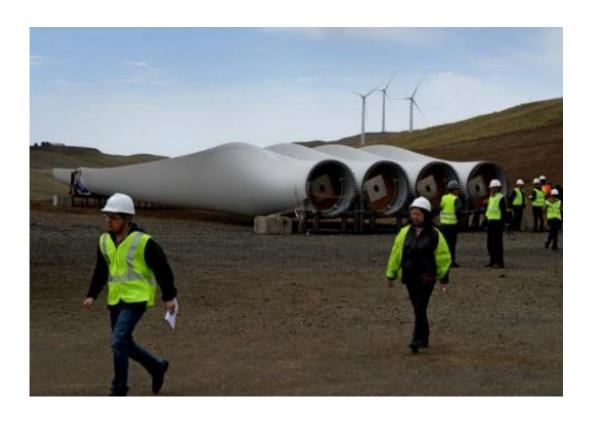
The blades of a soon-to-be-installed turbine at the Salkhit Mountain wind farm, 70 kilometres from Ulan Bator, June 4, 2013. A total of 31 turbines have been
