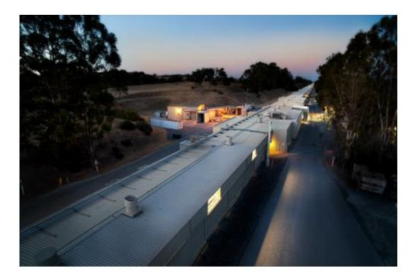
While SLAC's linear accelerator is in an underground tunnel, the power systems that help drive it are housed in this above-ground structure. A section of the linear accelerator is used to produce electron bunches that are converted to X-ray laser pulses for use in experiments at SLAC's Linac Coherent Light Source. Credit: SLAC Multimedia Communications
