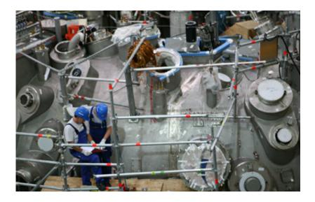
View of the Wendelstein 7-X fusion device from above: All of the 254 ports are installed. Credit: IPP, Anja Ullmann
