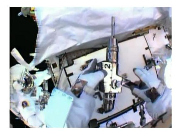
In this image made from video provided by NASA, astronaut Christopher Cassidy, foreground, holds a power wrench as he stows away a suspect coolant pump on the International Space Station on Saturday, May 11, 2013. Thomas Marshburn is at left. The two astronauts made the spacewalk to replace the pump after flakes of frozen ammonia coolant were spotted outside the station on Thursday. (AP Photo/NASA)
