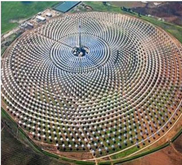
Gemasolar, a concentrated solar power plant in Spain.
