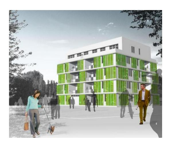
(Phys.org) —A 15-unit apartment building has been constructed in the German city of Hamburg that has 129 algae filled louvered tanks hanging over the exterior of the south-east and south-west sides of the
