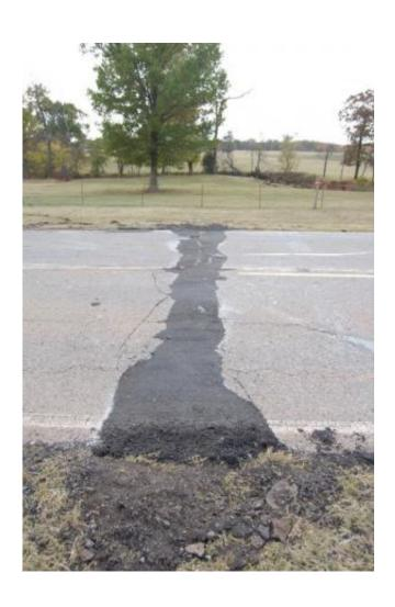
A 2011 magnitude 5.7 quake near Prague, Okla., apparently triggered by wastewater injection, buckled U.S. Highway 62. Credit: (ohn Leeman
