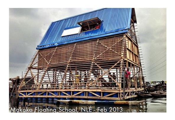
The Makoko Floating School is a three-story, 720-square-foot building afloat on a platform of recycled barrels and fitted with solar panels. The concept was the brainchild of forward-thinking Nigerian architect Kunlé Adeyemi. Credit: Kunlé Adeyemi
