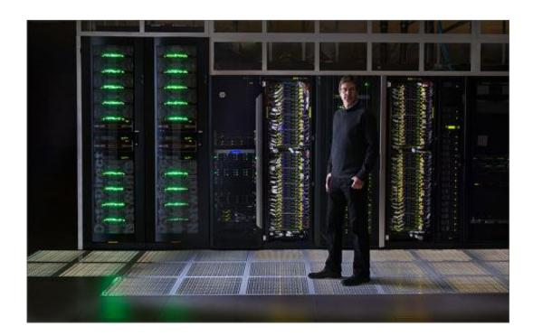
Steve Hammond, director of NREL's Computational Science Center, stands in front of air-cooled racks in the high performance computing (HPC) data center in the Energy Systems Integration Facility (ESIF). The rest of the system will be built out this summer using warm-water liquid cooling to reach an annualized average power usage effectiveness (PUE) rating of 1.06 or better. Credit: Dennis Schroeder
