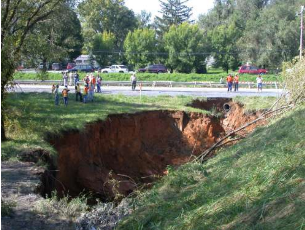
Sinkhole in Frederick, Maryland.
