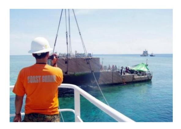
This photo, released on March 30, 2013 by Philippine Coast Guard (PCG), shows a portion of the stern of the USS Guardian being lifted by a boat crane during its salvage operation at Tubbataha reef, off Palawan island, western Philippines.
