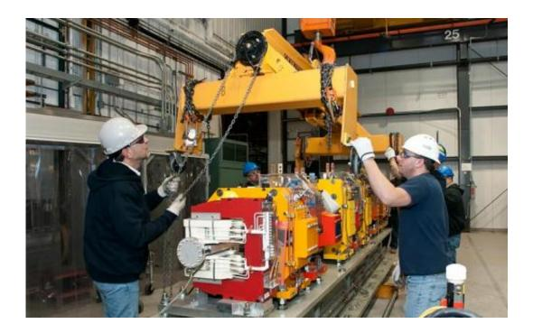
The final magnet girders are installed at Brookhaven's National Synchrotron Light Source II. Magnets traveled from across the globe, supplied by ring magnet vendors based in six countries: Buckley Systems Ltd (New Zealand), Budker Institute of Nuclear Physics (Russia), Danfysik (Denmark), Everson Tesla Incorporated (U.S.), Institute of High Energy Physics (China), and Tesla Engineering (U.K.).
