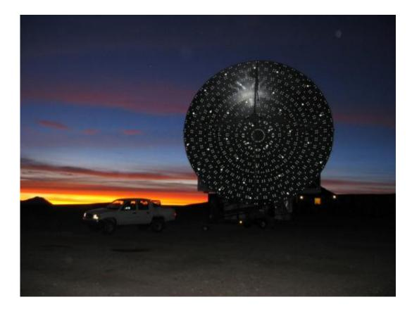
Pathfinder backlit by the sun just below the horizon at dusk: The Atacama Pathfinder Experiment had already begun operation in the Atacama Desert in Summer 2005. With an antenna diameter of 12 metres, it was the largest submillimetre telescope in the Earth's southern hemisphere. The camera flash is reflected off the adjustment screws of the individual panels, which permit the surface of the dish to be very precisely set. Credit: APEX
