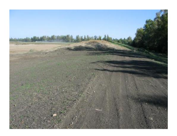
The original 60.5-foot Birds Point fuse plug was blown up using 265 tons of TNT on May 2, 2011. The USACE filled in the crater lake and temporarily patched the levee by putting in a patch that was 55 feet high in fall of 2011. In 2012 they restored it to the original height. Credit: University of Illinois
