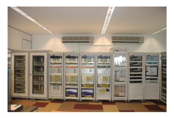
This is a Centre Tecnologic de Telecomunicacions de Catalunya ADRENALINE testbed showing a MPLS-TP access and aggregation network over a 4-node wavelength switched optical transport network. The multi-layer network can be controlled by either a distributed GMPLS control plane or an integrated stateful PCE/OpenFlow centralized control plane. Credit: CTTC Optical Networking Area, Spain
