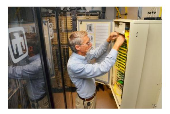
Steve Gossage, a senior engineer at Sandia National Laboratories, looks at fiber optics in a cable box that replaced heavier and bulkier copper cable for highspeed communications throughout much of the labs. Fiber offers more capacity and is more reliable than copper. Credit: Randy Montoya
