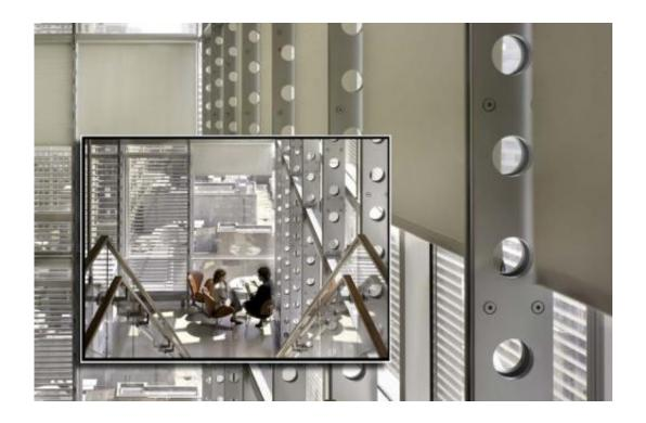
To control daylighting for maximum comfort and energy efficiency, computercontrolled shades respond to changing exterior conditions. Credit: Renzo Piano Design Workshop
