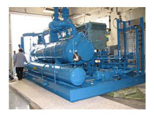
A compressor being installed for the new 20 Kelvin helium refrigerator at NASA Johnson Space Center's Space Environment Simulation Lab Chamber A. The new system will allow testing of components of the James Webb Space Telescope.
