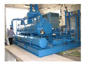
A compressor being installed for the new 20 Kelvin helium refrigerator at NASA Johnson Space Center's Space Environment Simulation Lab Chamber A. The new system will allow testing of components of the James Webb Space Telescope.
