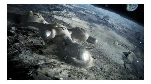
Multi-dome lunar base being constructed, based on the 3D printing concept. Once assembled, the inflated domes are covered with a layer of 3D-printed lunar regolith by robots to help protect the occupants against space radiation and micrometeoroids. Credit: ESA
