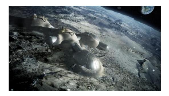
Multi-dome lunar base being constructed, based on the 3D printing concept. Once assembled, the inflated domes are covered with a layer of 3D-printed lunar regolith by robots to help protect the occupants against space radiation and micrometeoroids. Credit: ESA
