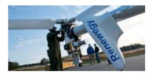
An offshore wind test turbine has been erected behind the University of Maine Advanced Structures and Composites Center on campus to evaluate sensor systems and controls in preparation for the installation of a floating turbine in the Gulf of Maine this spring as part of the DeepCwind Consortium project.
