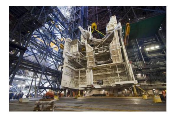
As part of NASA's Ground Systems Development and Operations Program, a space shuttle-era work platform is being moved to the floor high bay 3 of the VAB. GSDO is developing the ground systems, infrastructure and operational approaches to safely process, the next generation of rockets and spacecraft. Credit: NASA/Jim Grossmann
