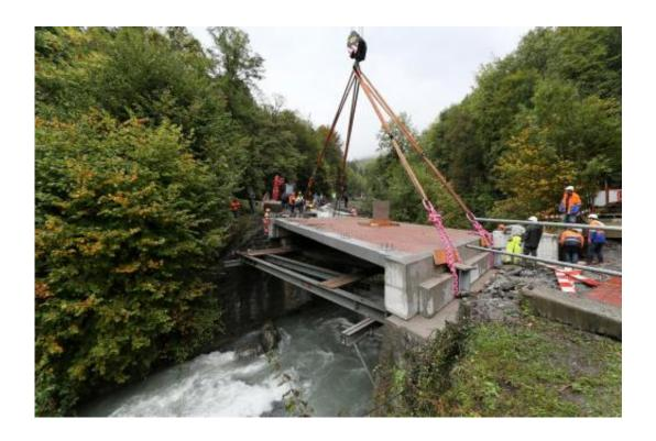
A bridge with a balsa wood core was built in Bex, Switzerland. The prefabricated bridge deck was mounted in a single day. Credit: 2012 EPFL - Alain Herzog
