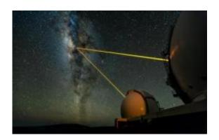
The two W. M. Keck Telescopes on Mauna Kea, Hawaii, observing the galactic center. The lasers are used to create an artificial star in the Earth? supper atmosphere, which is then used to measure the blurring effects of the lower atmosphere (the effect that makes the stars twinkle in the night sky). The blurring gets corrected in real time with the help of a deformable mirror. This is the adaptive optics technique. Credit: Ethan Tweedie
