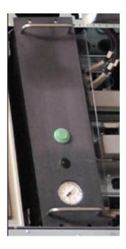
Cool-Flo pump, with simple stop/start interface, is conveniently located uder the server rack for easy access.
