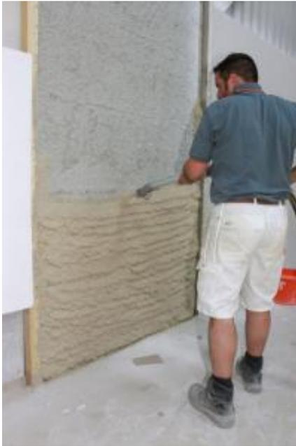
(Phys.org) -- Old buildings are beautiful – and hard to insulate. Empa and the Swiss render manufacturer Fixit AG together developed a new Aerogel-based plaster that provides twice the insulation of currently used insulating renders. The product should come onto the market next year.
