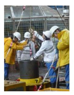
This shows the researchers running the sensor array into tubing. Credit: JAMSTEC/IODP, photo taken by Jim Mori
