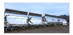
Parabolic trough collectors at the PSA, Plataforma Solar de Almeria, experimental facilities in Spain. Concentrated sunlight heats up a synthetic oil in the pipes at the focus of the troughs. Photo: Erik Pihl
