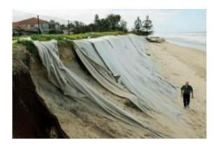
Felt sheeting is seen draped over sandhills to help slow the progress of erosion in front of the Meridien holiday apartments at Old Bar Beach at the coastal town of Old Bar in Australia's New South Wales state. Old Bar is the most rapidly eroding and at-risk piece of coast in populous New South Wales state, losing an average one metre of seafront every year.
