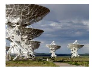
The Jansky Very Large Array radio astronomy telescope array consists of twenty-seven, 230-ton, 25-meter diameter dish antennas that together comprise a single radio telescope system. Credit: National Radio Astronomy Observatory
