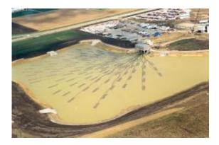
Geothermal coils are visible in a partially filled heat rejection lake at the Great River Medical Center in Burlington, Iowa. For buildings that are predominantly in cooling mode, lake source geothermal can provide substantial energy savings. Credit: KJWW Engineering Consultants
