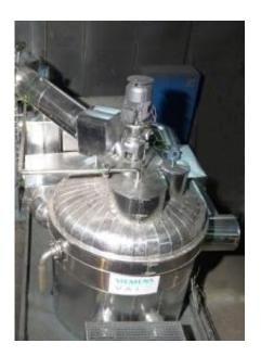
Heat recovery plant installed by Siemens in the electric steel plant of Stahlwerk Thüringen GmbH in Unterwellenborn (Germany). The pilot plant runs with molten salt, and is used for material validation and process optimization.
