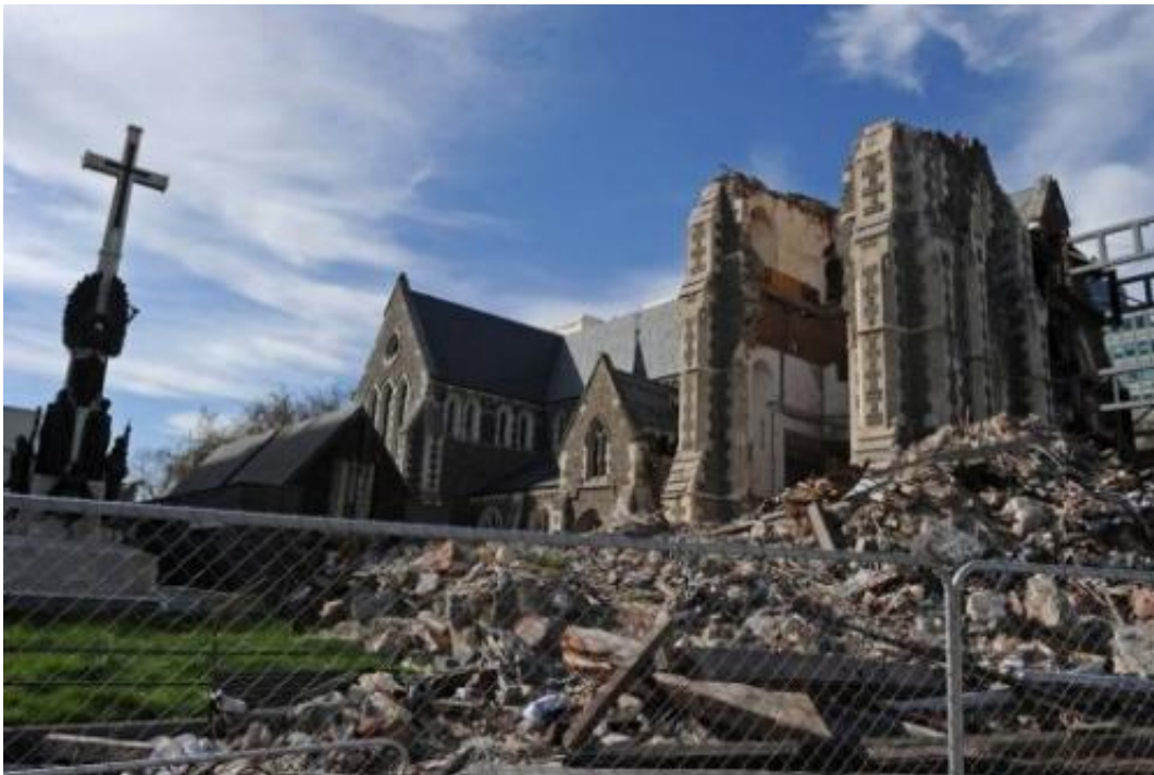
File photo shows the damaged Christchurch Cathedral in the New Zealand South Island city of Christchurch in September 2011. The 6.3-magnitude quake that
