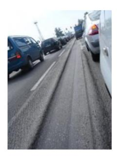
Ruts like these pose a serious threat to motorists. Zhanping You and his team have discovered that adding nanoclay to the asphalt pavement mix may help roads resist rutting.
