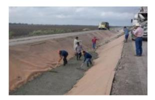
Workers in Hidalgo County spread concrete over a synthetic canal liner made of polyester. Credit: Texas AgriLife Extension, Askar Karimov
