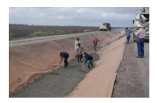
Workers in Hidalgo County spread concrete over a synthetic canal liner made of polyester. Credit: Texas AgriLife Extension, Askar Karimov
