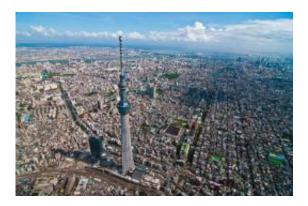
The world tallest (634 m) sightseeing and TV broad casting tower - Tokyo Sky Tree uses a massive amount of most advanced TMCP steels. Credit: STAM
