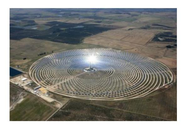
The Torresol Energy Gemasolar plant in Fuentes de Andalucia near Seville. The unique thermosolar power station in southern Spain can shrug off cloudy days: energy stored when the sun shines lets it produce electricity even during the night.
