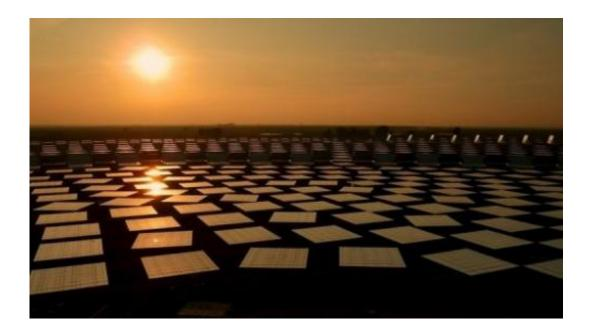
It is the station's capacity to store energy that makes Gemasolar so different because it allows the plant to transmit power during the night, relying on energy it has accumulated during the day.
