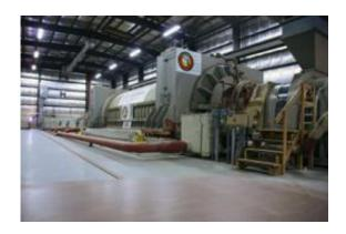
The 1,200-megajoule motor generator that powers the magnetic pulse.
