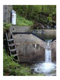
This is an image of a weir used to monitor stream flow patterns in the Hubbard Brook Experimental Forest. Credit: Cary Institute Photo Archive.
