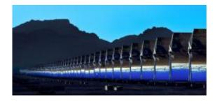
Abengoa is erecting more than 3,200 mirrored parabolic troughs at its Solana plant near Gila Bend, Ariz. When at full operation, the CSP plant will serve more than 70,000 homes. Credit: Dennis Schroeder
