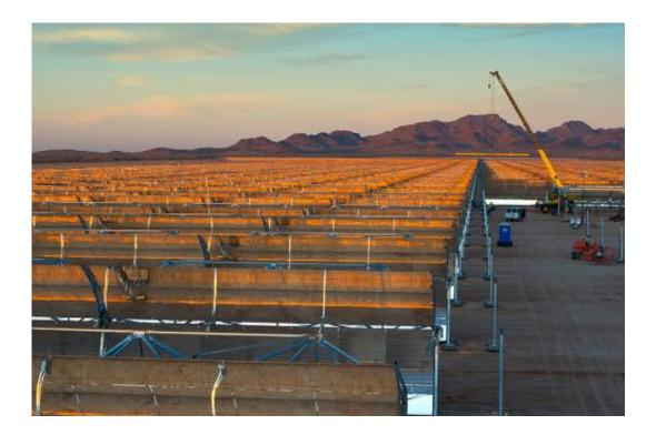
Crews work around the clock installing mirrored parabolic trough collectors built on site — that will cover 3 square miles at Abengoa's Solana Plant. When finished, the plant will generate 280 megawatts of clean, sustainable power. Credit: Dennis Schroeder
