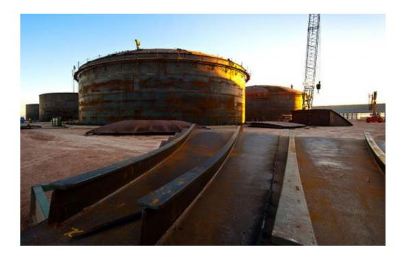
The tanks that hold the molten salts at Abengoa's Solana Plant are enormous. The salts can keep the solar-heated fluids very hot for several hours, so they can be transferred to turbines to produce electricity even when the sun isn't shining. Credit: Dennis Schroeder
